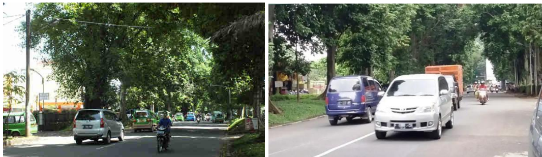
Figure 5.10. Condition of Dr. Sumeru Road
